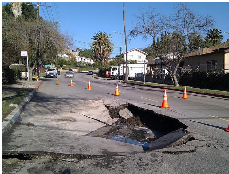
Figure 4-48. Subsidence example in San Joaquin Valley.
