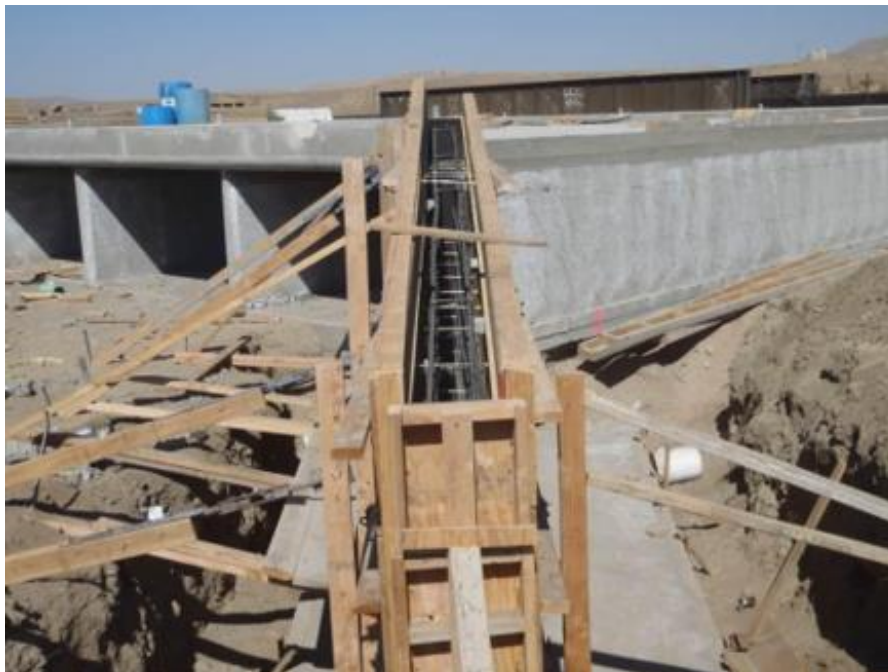
Figure 2-3: Bena Bridges During Construction
